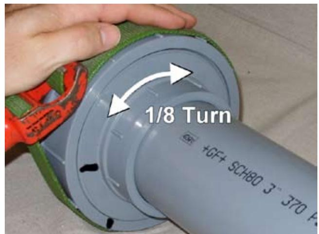
At this point, the system should be hydrostatically pressure tested before turning the union nut any farther.
